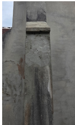
Exposed brick visible due to deteriorating stucco
